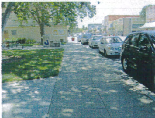
Public right of way North First Street- Needs directional access signage
