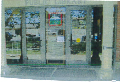
Entry door compliant. Provided with auto-door opener
