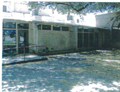
Rear courtyard access points from building
