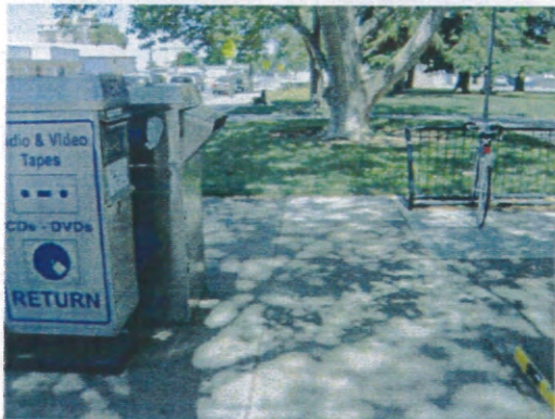
Book drop access compliant for running and cross slope, path of travel access and reach height
