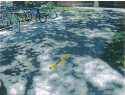
Access from public right of way compliant for running and cross slope
