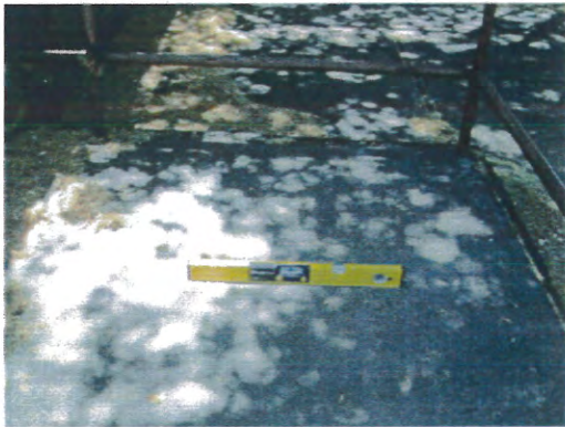
Ramp Landing cross slope compliant
