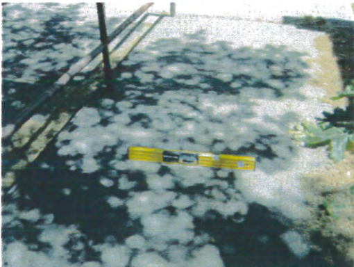
Ramp cross slope compliant at less than 2%
