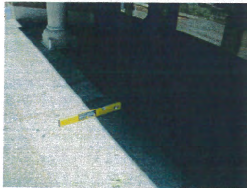
Landing running and cross slope compliant
