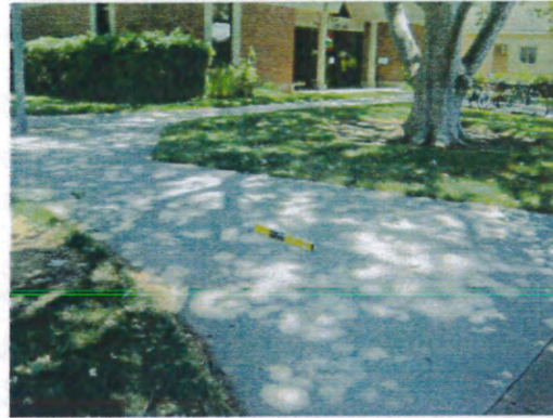
Access from public right of way compliant for running and cross slope
