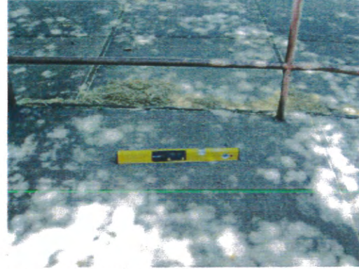
Landing running slope compliant
