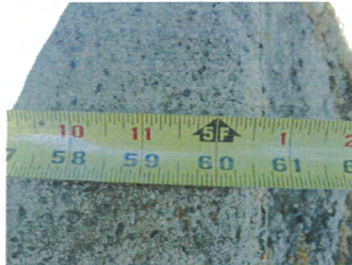
Ramp width compliant at more than 48"
