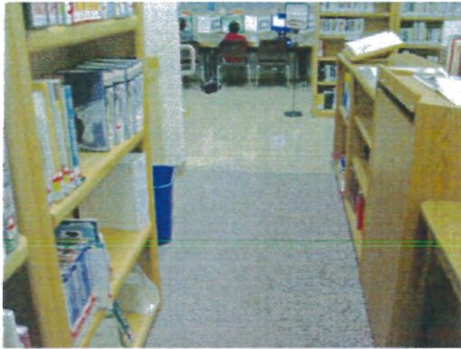
Access aisle to print station. End aisle compliant at 36"
