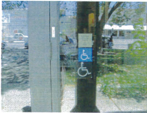
Entry door compliant. Provided with auto-door opener
