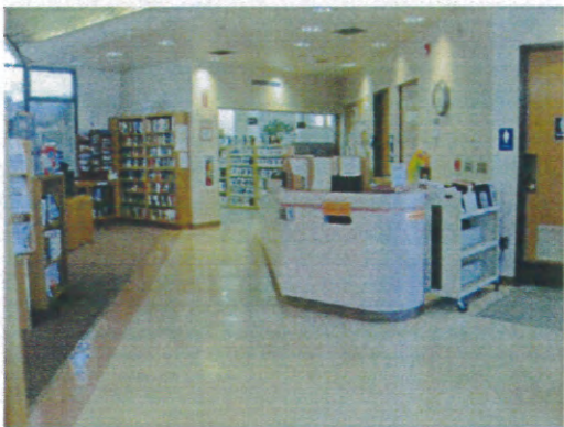
Library Service Counter compliant for height and path of travel access
